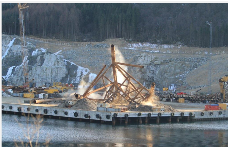
Figure 3: Example of dust escape when platform structures are tipped over.
