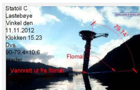
Figure 18: 79.74° tilting of Statfjord C loading buoy
