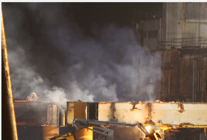
Figure 4: Example of dust escape due to torch cutting.
